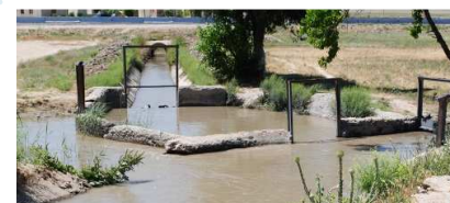
Water distribution structure, Samarkand province (photo is taken by project)
