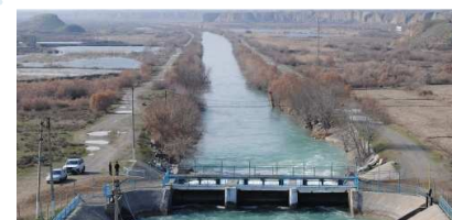
Canal Eski Anchor, Samarkand province (photo is taken by project)
